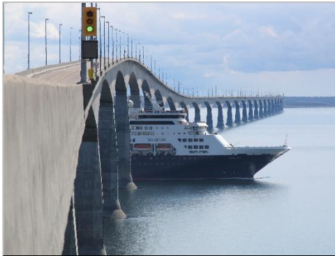
Confederation Bridge and Ferry Source: Strait Crossing Bridge Limited
